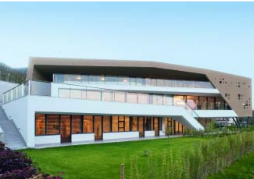
With its protective concrete encasement, the spacious two-unit apartment building bows before the terrors of the surrounding vineyards.
