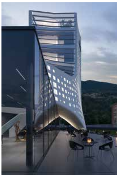
Neubau Durst Phototechnik AG, Brixen, (monovolume architecture + design, 2019)
